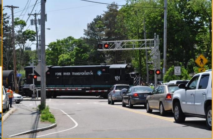
*Commercial Street At-Grade Crossing in Braintree, MA with Flashing Lights and Four-Quadrant Gates*
