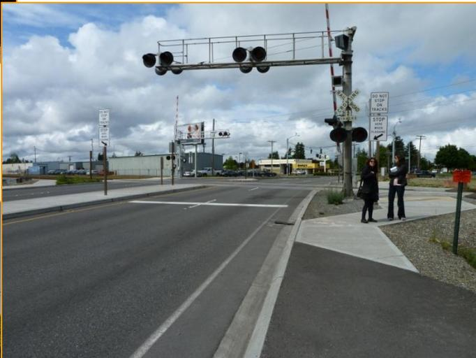
*100<sup>th</sup> Street At-Grade Crossing in Lakewood, WA Upgraded with Center Curb Median, Wayside Horns, and Flashing Lights and Gates*
