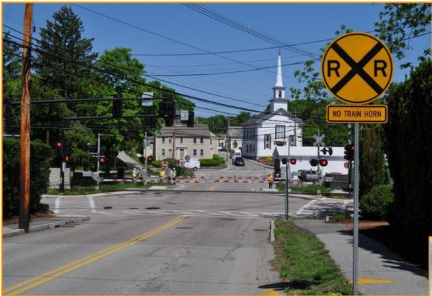
*A Four-Quadrant At-Grade Crossing Intertied with a Traffic Signal in a Quiet Zone at Hersey St., Hingham, MA*
